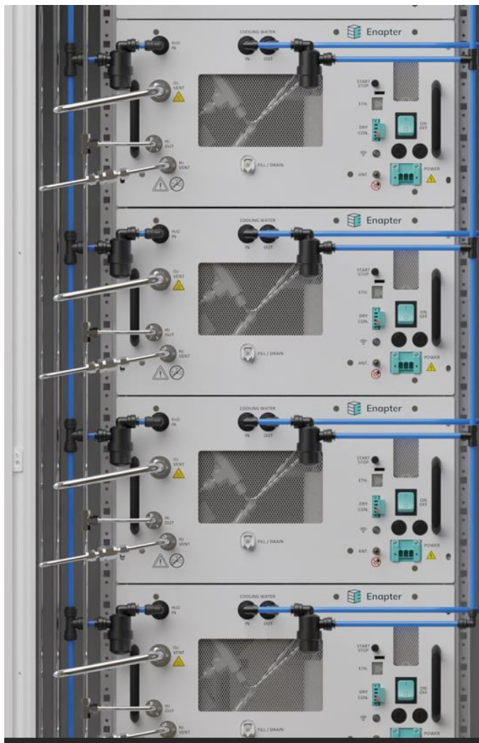
Three EL4.1 with common H 2 OUT connected to a DR2.1 <5>
